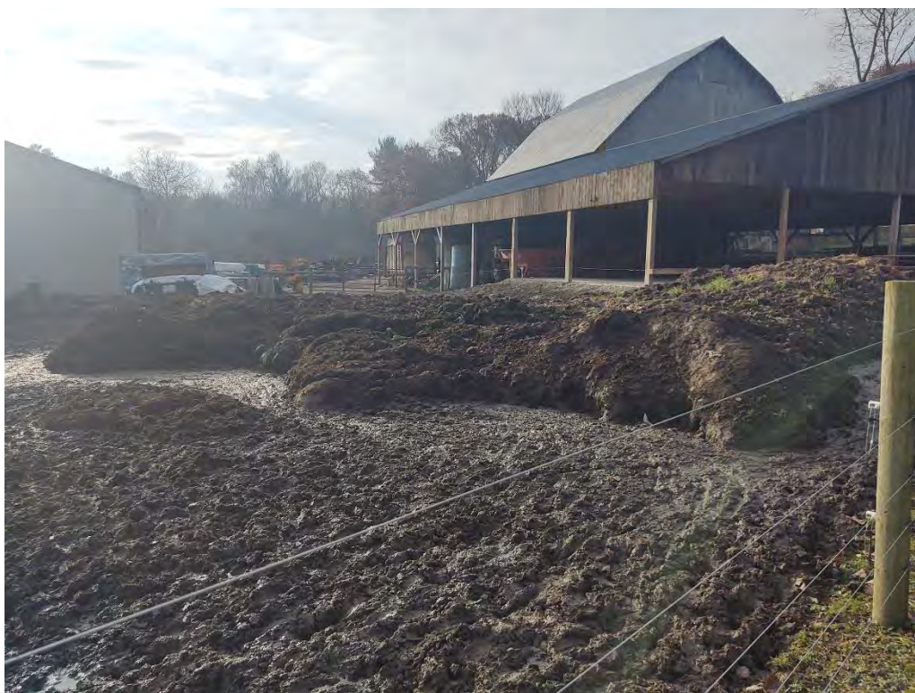
Manure stacked outside, earthen feedlot. Recent addition to bank barn seen here: "Barn #2"
