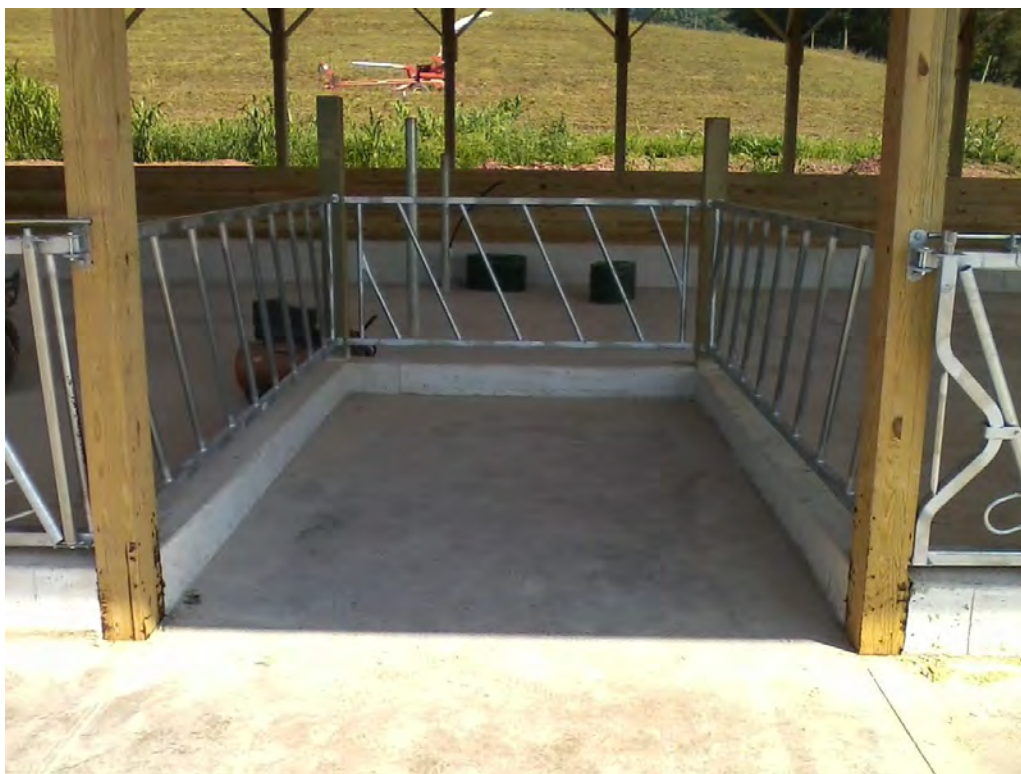
Picture of Built-in-FeedBunk Perpendicular to Building: open to eave-side
