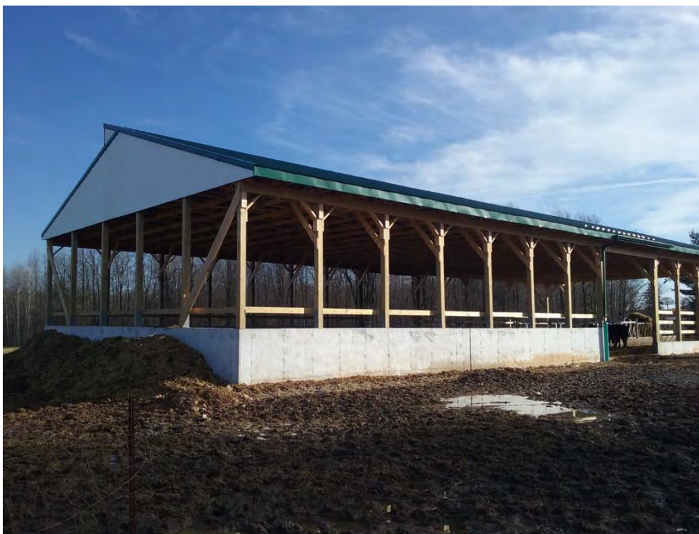
Example: Picture of manure stacking building with posts on top of walls
