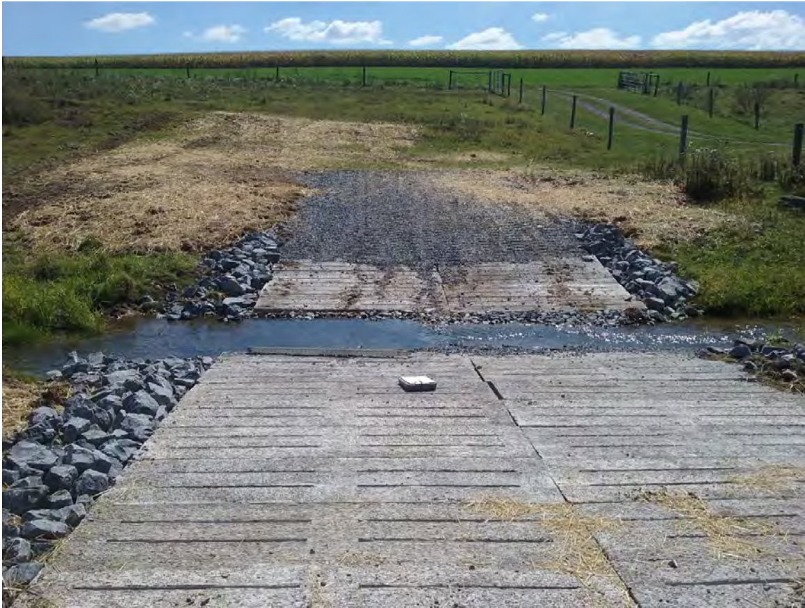
Example Stream Crossing with Pre-cast Slats, Rip-Rap Frame and Gravel Approach
