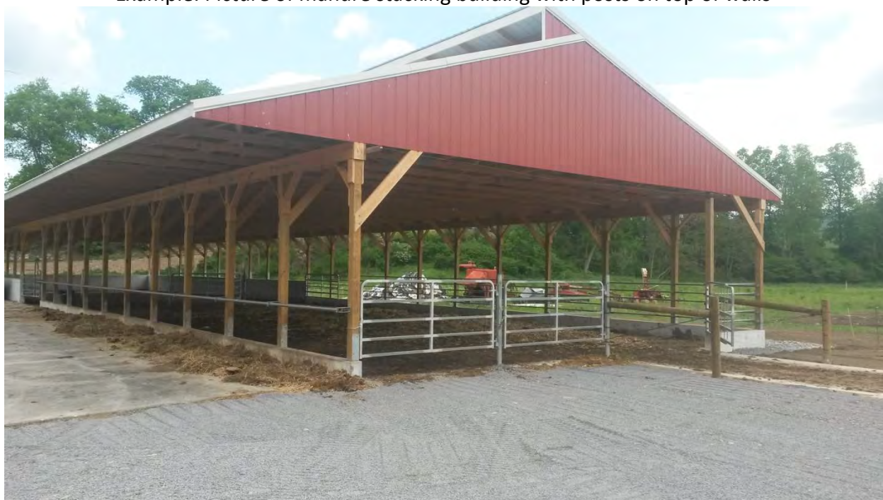
Example: Combined Roofed Feedlot with Manure Stacking Area in the rear of building With 8' overhang for drive-by-feeding
