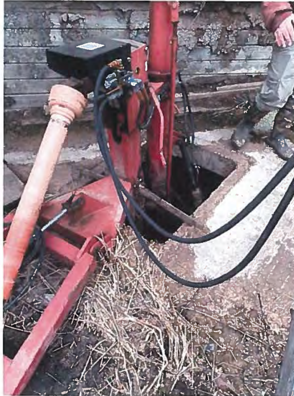
EXISTING PUMP/RECEPTION PIT
