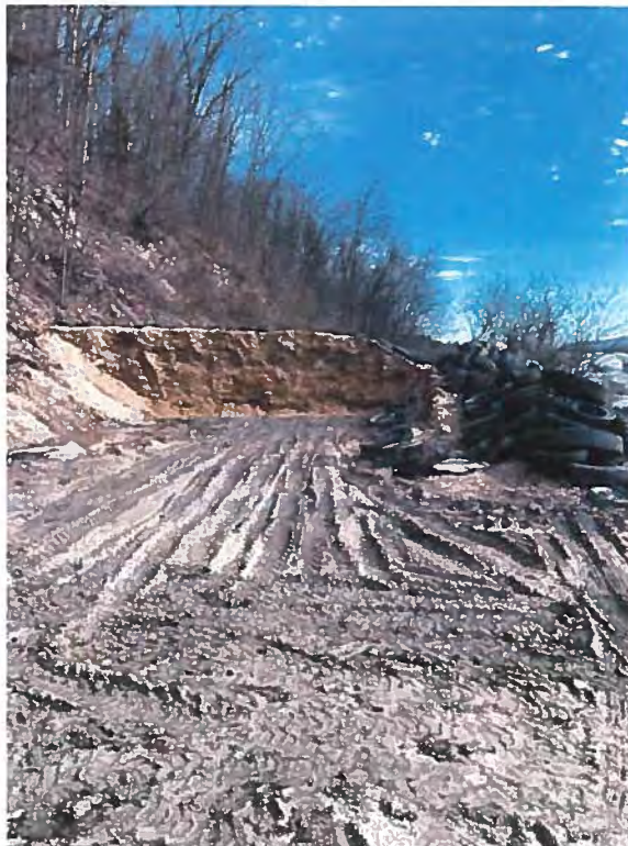
EXISTING BUNK SILO
