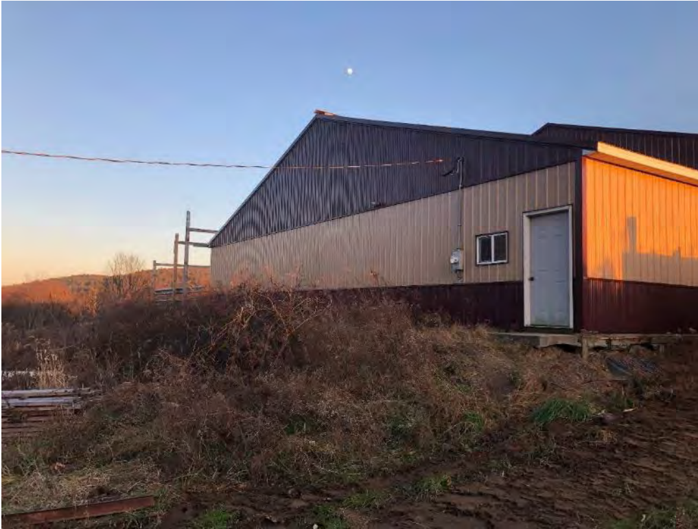
1 - North end of beef barn where manure stacking area is planned.
