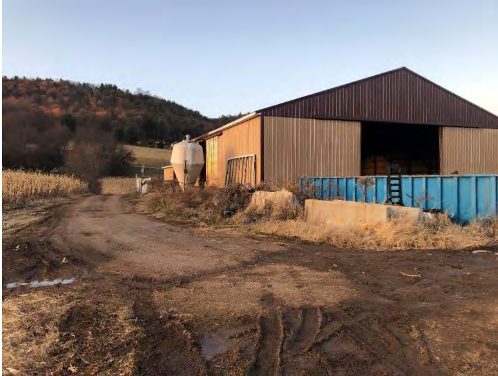
3 – South end of barn.
