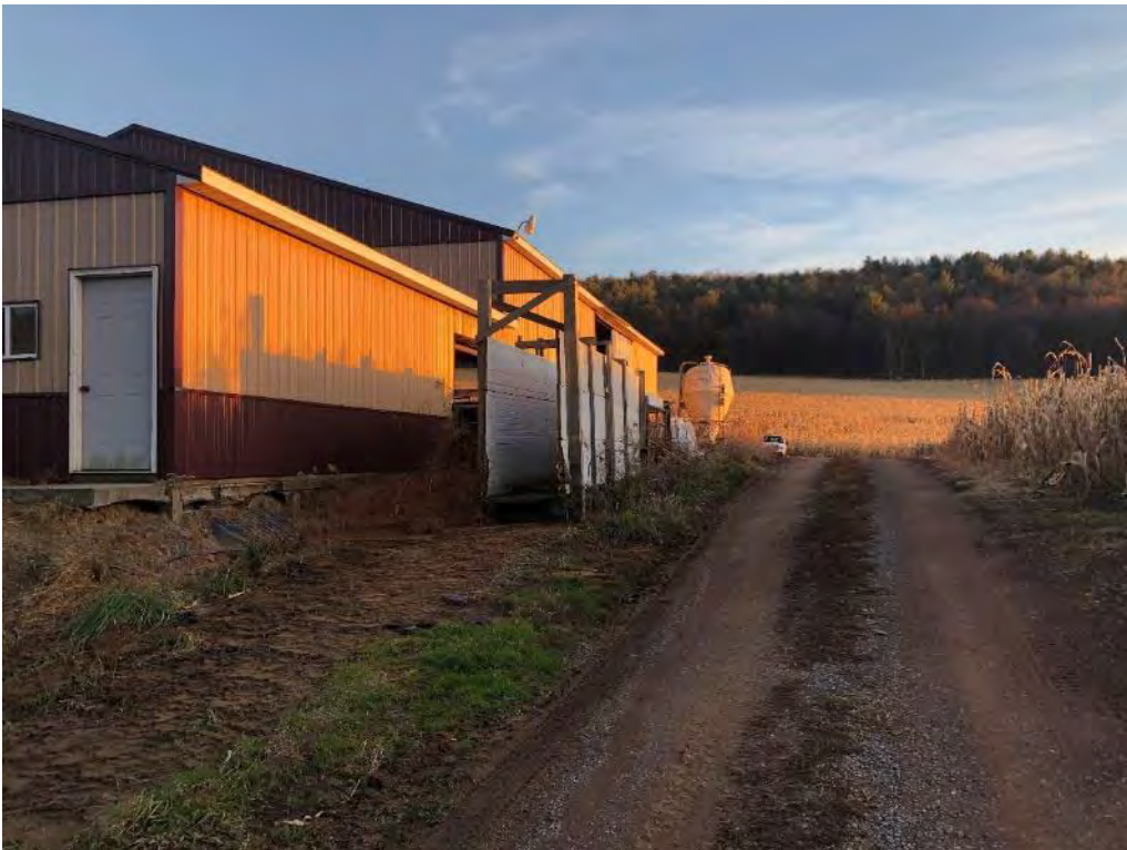
2 - West side of barn.
