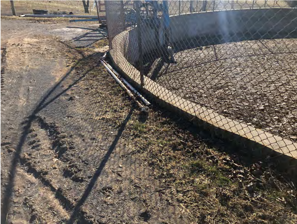
10 – Concrete manure storage at dairy barn.
