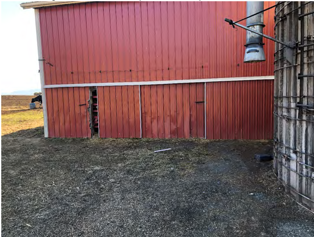
8 – Silo loading area. Concrete HUAP planned here to prevent erosion.
