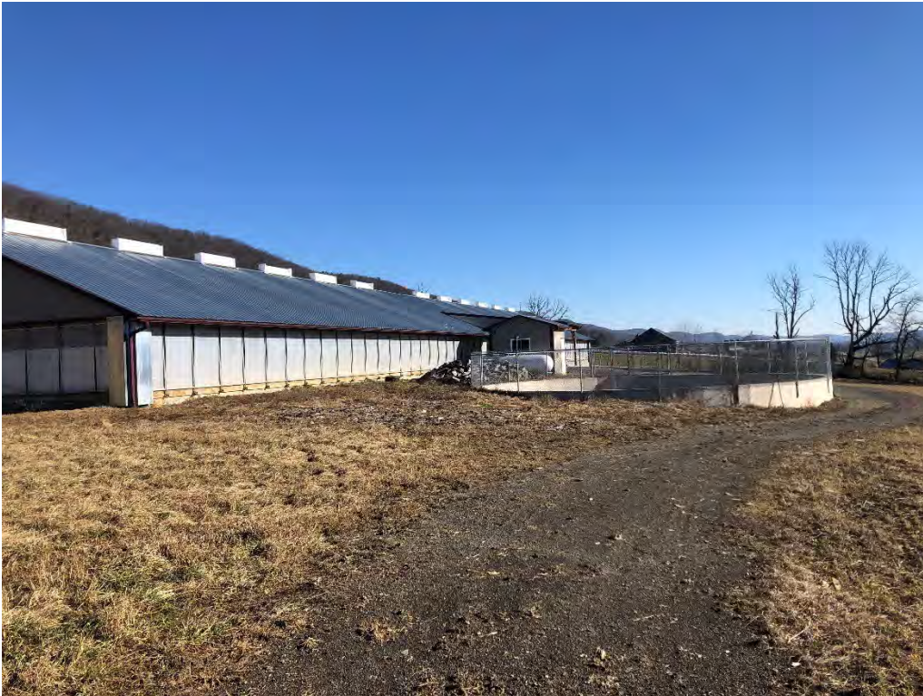
12 – Existing manure storage at veal barn (HQ2) – looking east.
