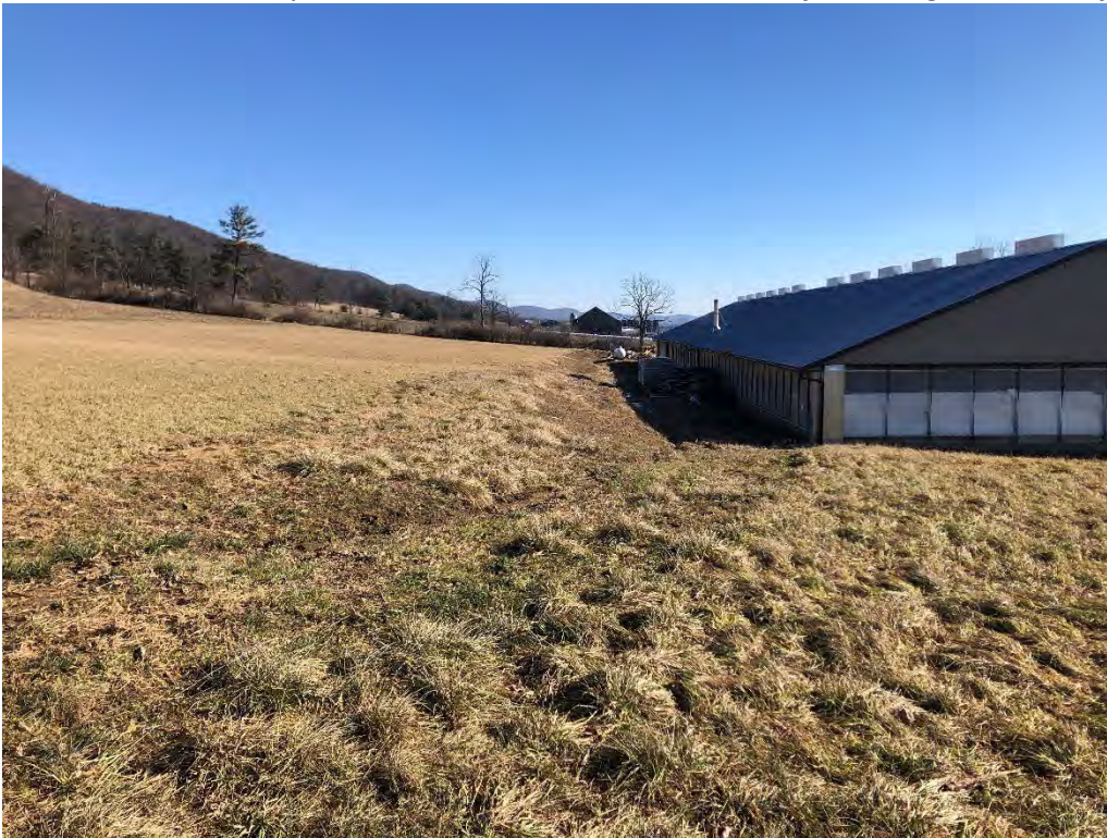
14 – Grassed waterway to outlet here. Water will continue to flow along north side of veal barn.
