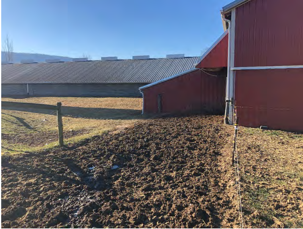
7 – This section of walkway from dairy barn is concrete..
