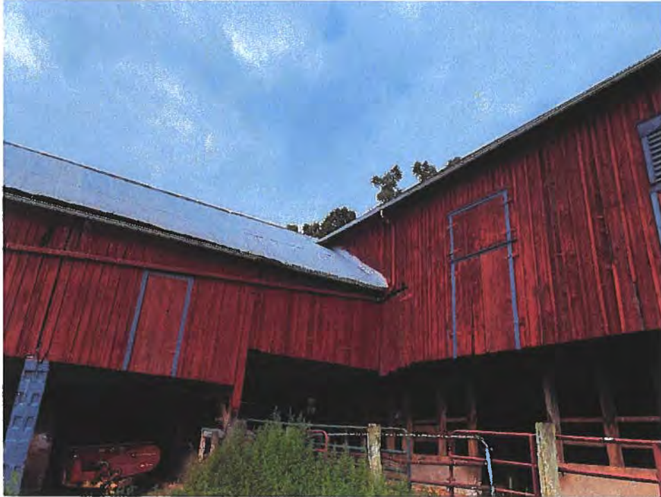
ROOF LINES OF EXISTING BARN
