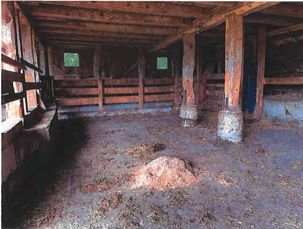
INSIDE OF EXISTING BARN
